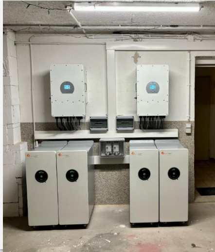
24kW/50kWh Hybrid ESS of PV&DG (Diesel Generators)
